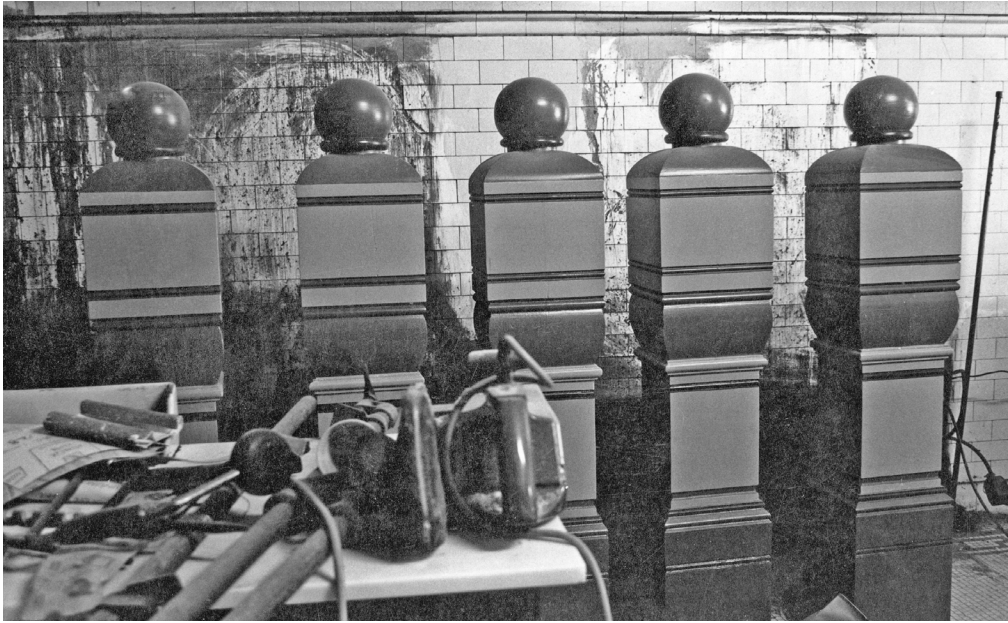
Figs. 2a–b. Above: Posts built by Moore to replace older versions in Pullman, Illinois; his tools in foreground and the greasy wall from restaurant cooking in back. Right: New post and rail installed in Pullman. Photographs courtesy Timothy Moore, 1977.
